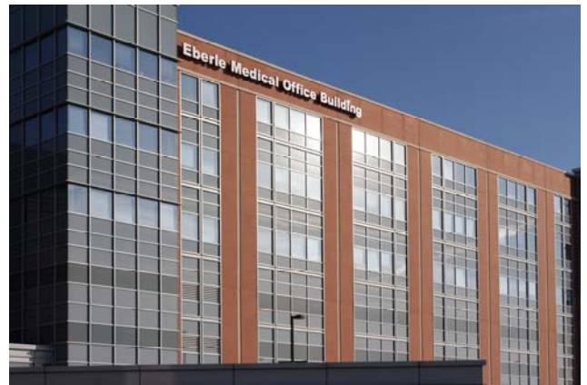
Eberle Medical Office Building Alexian Brothers Medical Center – Elk Grove Village, IL
